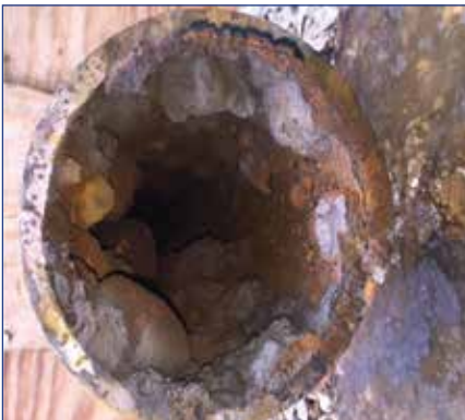
Before: Huntingburg's 120 year old pipe prior to cleaning and lining
